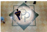
Water jet or laser technology used to inset logos into porcelain tiled field.
