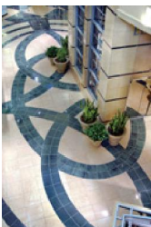
Custom laser cut curvilinear tile patterns are repeated at different scales. The border curves and meanders throughout the entire length of the wall.
